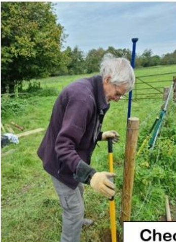
Digging footings for metal gate frame
