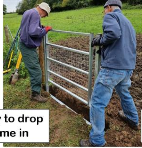
Mixing ballast with cement and squaring up the gate
